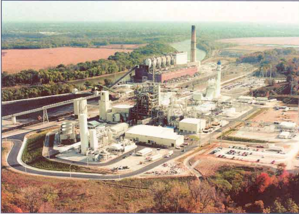
The Wabash River Coal Gasification Repowering Project
